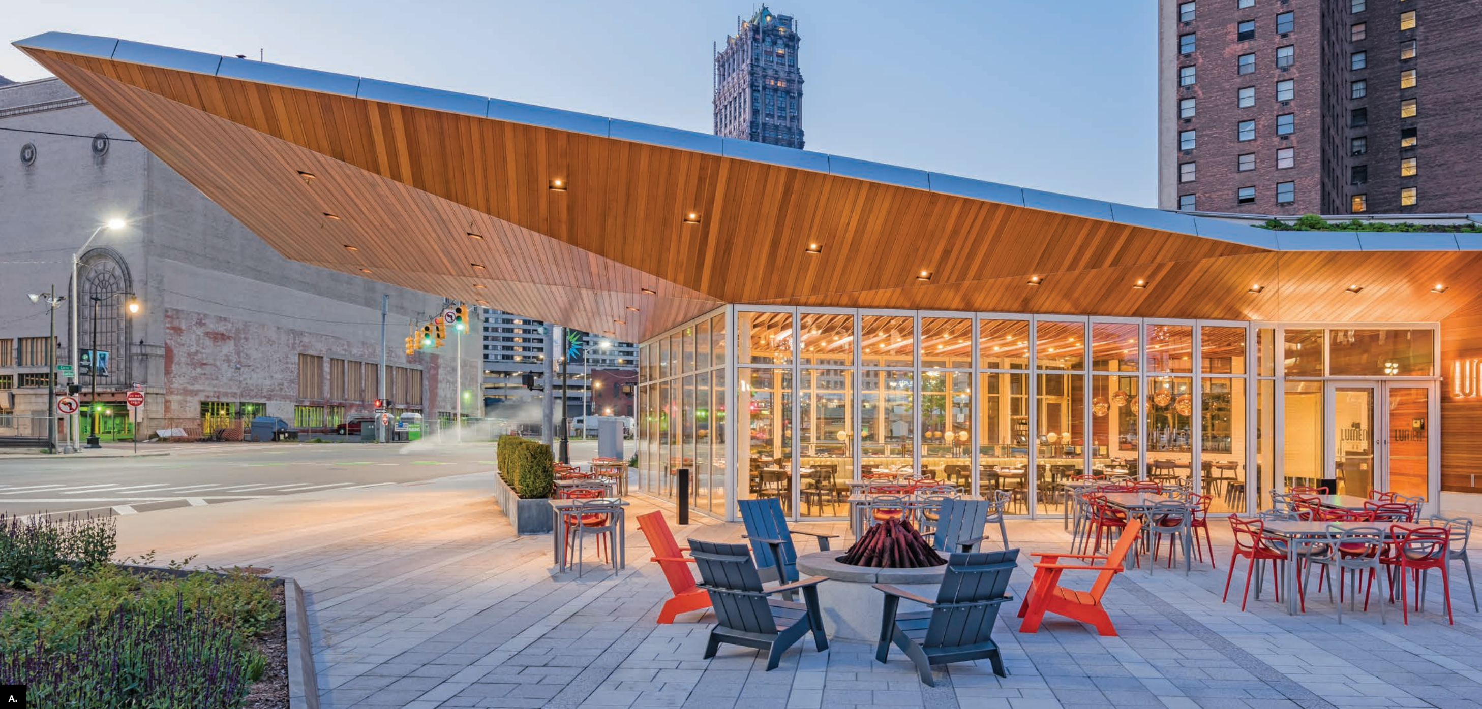
A. Lumen Restaurant, Detroit MI HSW60, panels stack within opening, weather resistant low profile no channel saddle sill, open corner configuration Architect: Touloukian Touloukian, Inc. Glazing Contractor: Edwards Glass Company
